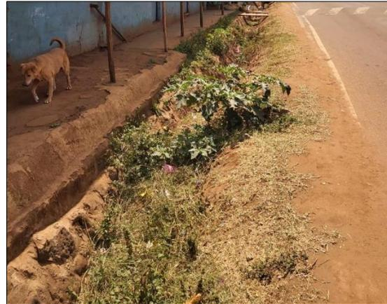
**Plate 7: Open Storm Water Drainage System**
